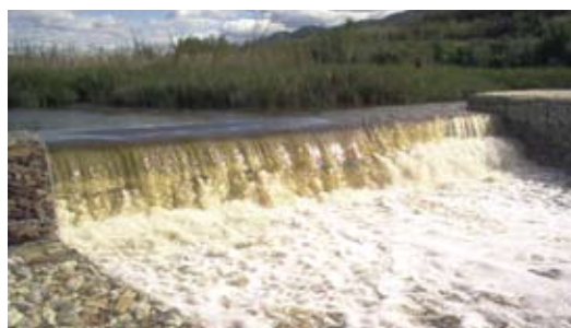
A retaining weir, built by Working for Wetlands, reduces erosion of a montane stream during summer flooding.
