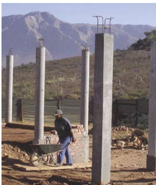
Construction begins on the new tearoom in the Karoo Desert NBG.
