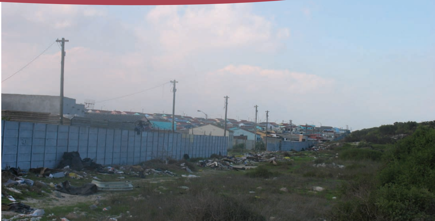
Charline feels that this vibracrete fence has created more problems than solutions
