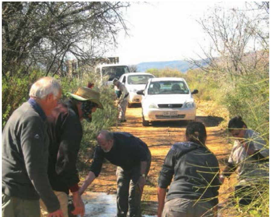
Outramps face many challenges in their quest for monitoring. Here they are re-building roads to cross a river.
