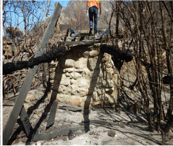
Fig 2 - Stone masonry abutment
