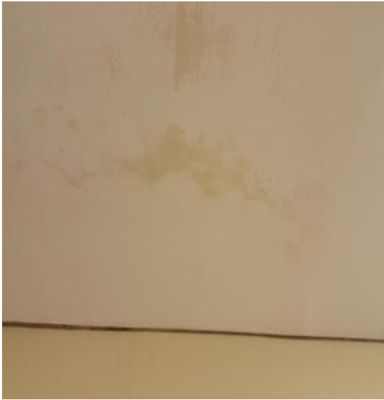
Fig.1. Water ingress due to leaking box gutter Fig.2. Box gutter
