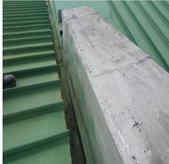
Fig.1. Water ingress due to leaking box gutter Fig.2. Box gutter
