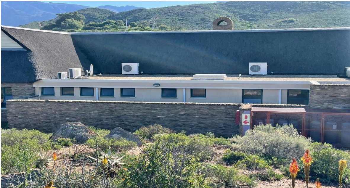
Fig 3. Restaurant concrete roof
