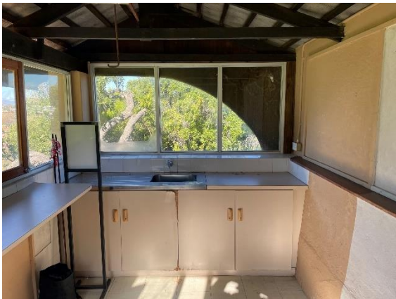
Fig 1. Replace existing sink cabinet
