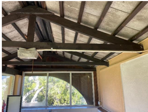
Fig 2. Roof trusses and light fitting
