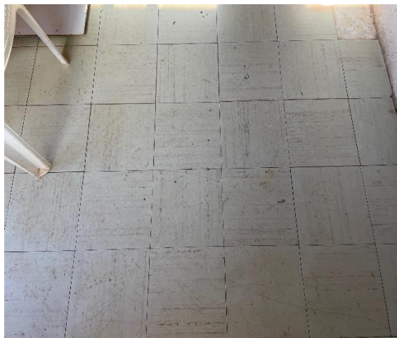
Fig 6. Existing vinyl floor tiles
