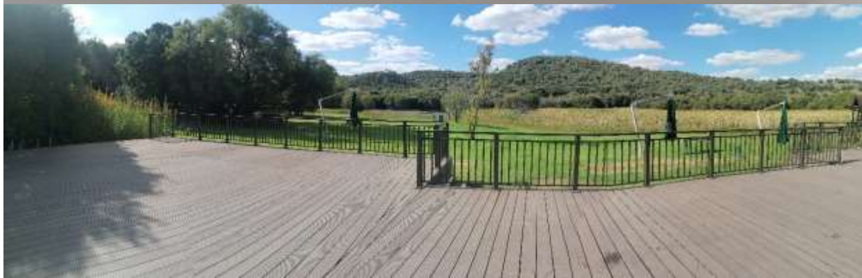
Picture of the newly constructed deck
