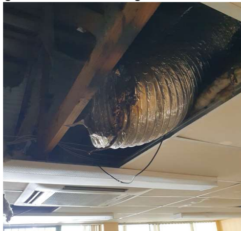
Figure 2-9: HVAC&R damages
