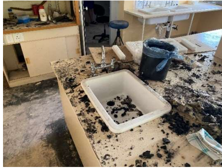
Figure 2-15: Alteration to work tops
