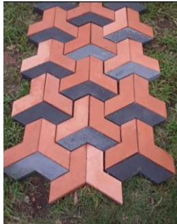
Coble bond paving
