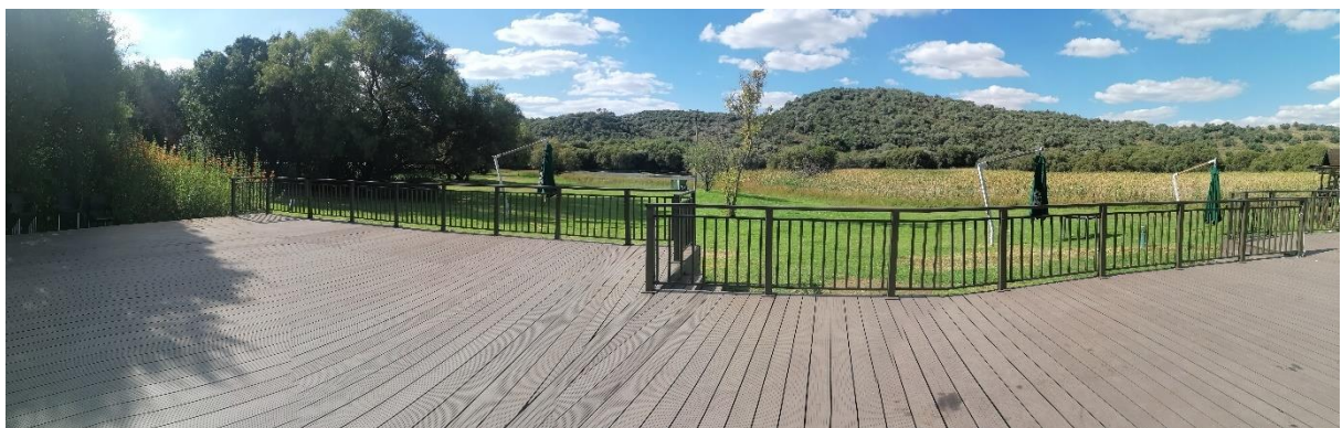
Picture of the newly constructed Deck
