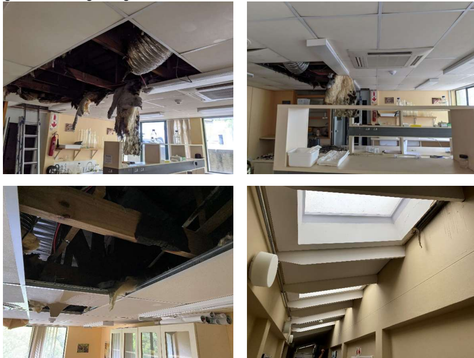
Figure 2-11: Ceiling damages
