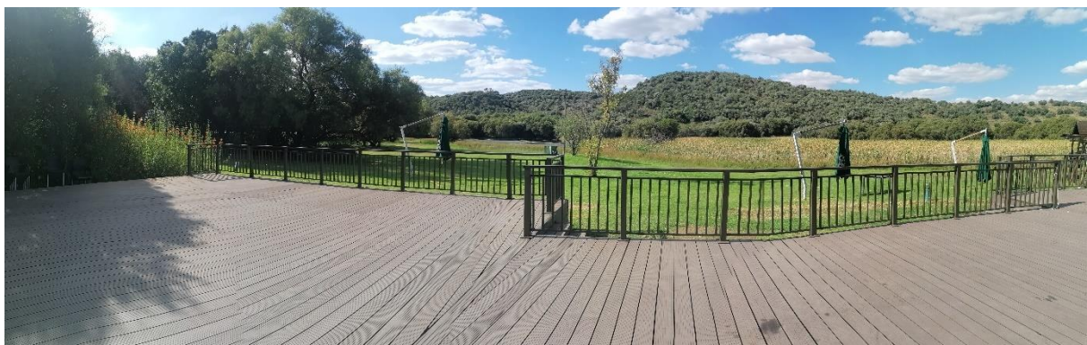
Picture of the newly constructed Deck
