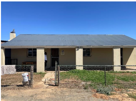
Fig 1. Front view of house
