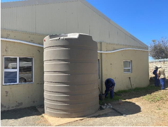
Fig 3. Extent of external damp wall
