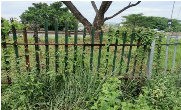
Fig 3: Palisade fence that needs painting maintenance
