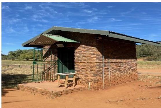
Fig. 3: External view of guard house
