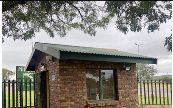
Fig. 2: External view of guard house
