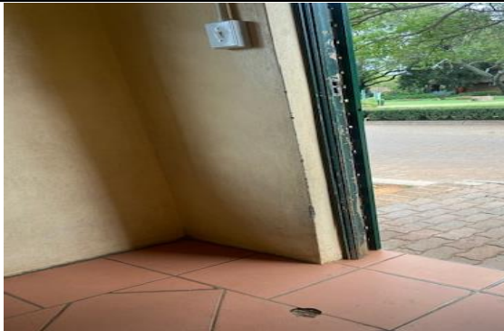
Fig. 1: Existing internal floor tiles
