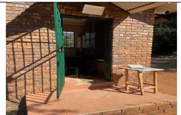
Fig. 4: Existing internal and external tiles
