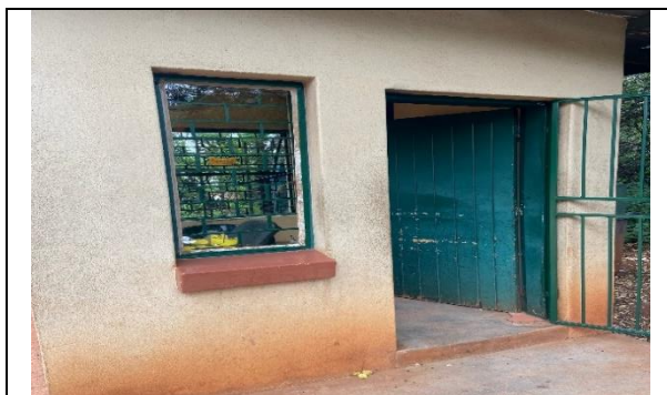
Fig. 5: External view of guard house
