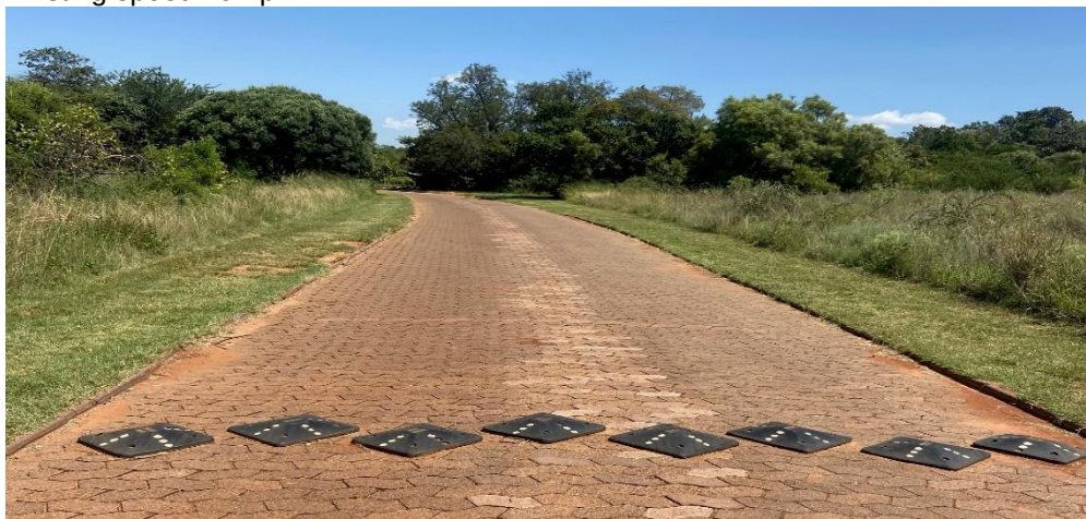
Existing speed hump
