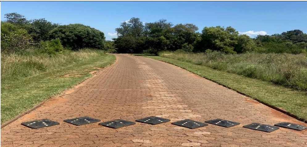
Fig. 2: Existing rubber speed humps 50mm (H)
