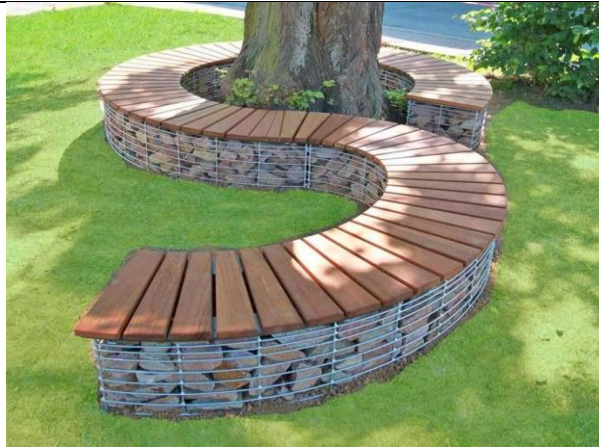
Fig. 1: S-shape gabion bench
