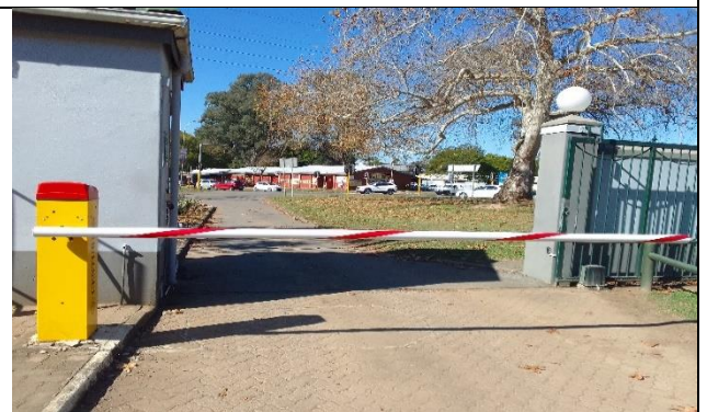
Fig.6: Existing Entrance boom gate
