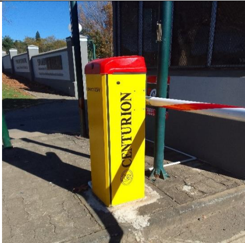
Fig.3: Existing centurion boom gate system box
