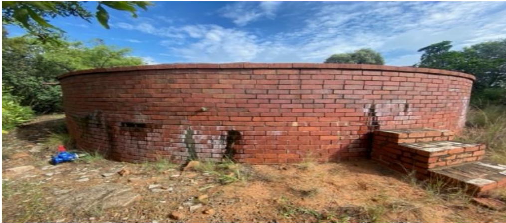
Fig.2: Existing finishes of reservoirs
