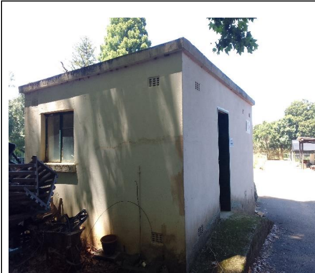
Fig.1: Chemical Store building
