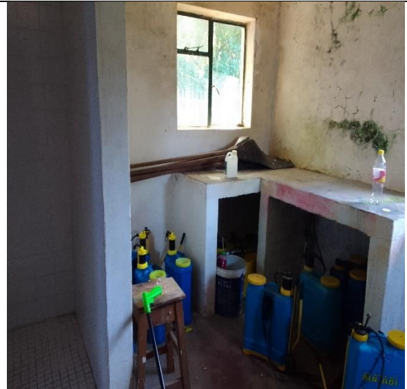
Fig.6: Room to be repaired
