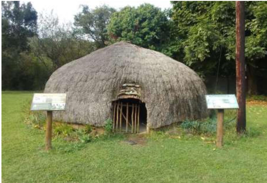
A thatched hut requiring repairs
