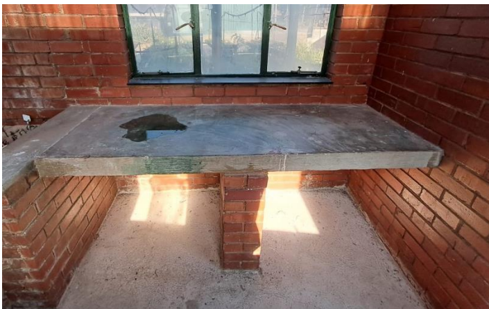
Image 2 : Typical work bench made of brick and concrete
