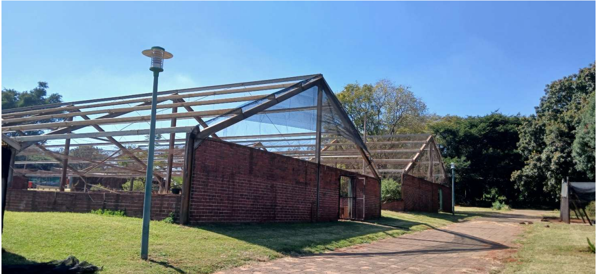
Figure 1: Picture of the two Nurseries to be renovated from the outside
