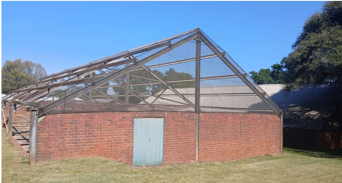
Figure 5: Shows existing doors
