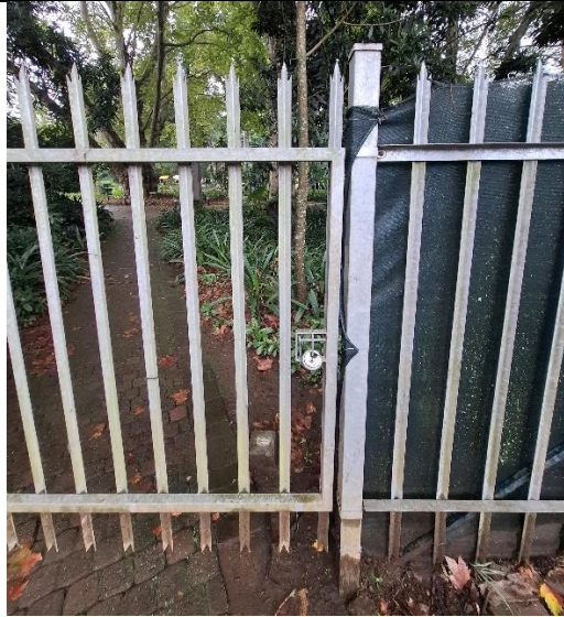
Fig.1: Existing staff gate with a padlock
