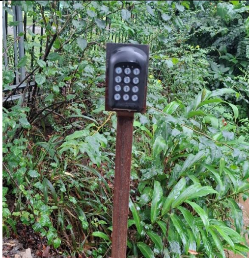
Fig.5: Example of the required Keypads for the existing gate motor
