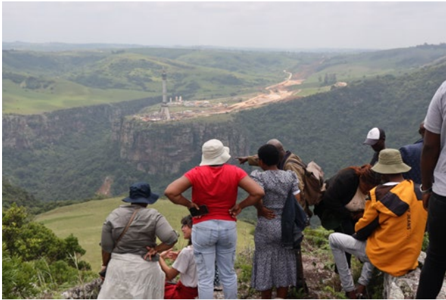
The Msikaba bridge, currently under construction, forms part of the N2 Wild Coast Road project and aims to improve the travel time between Durban and East London for light and heavy freight vehicles.
