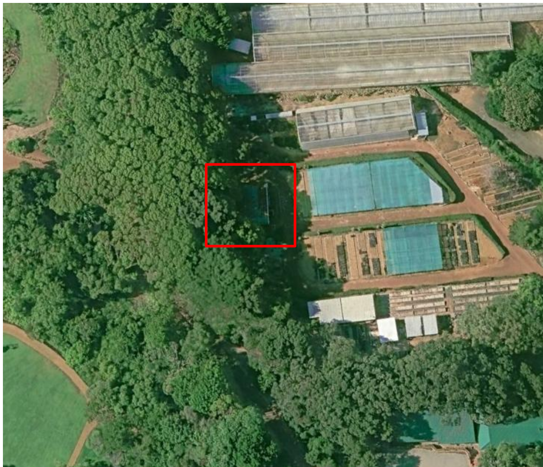
Figure 1: Nursery Building N33 Locality
